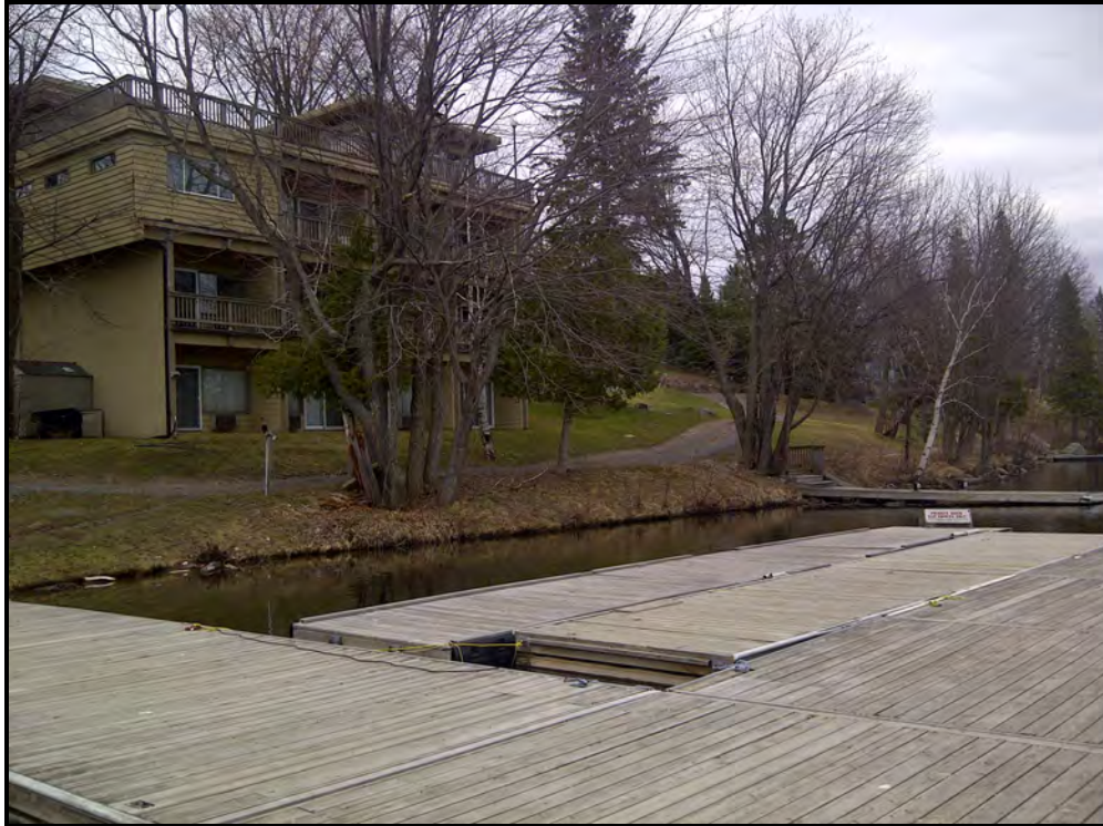
Figure 5 – Existing Terrace Building
